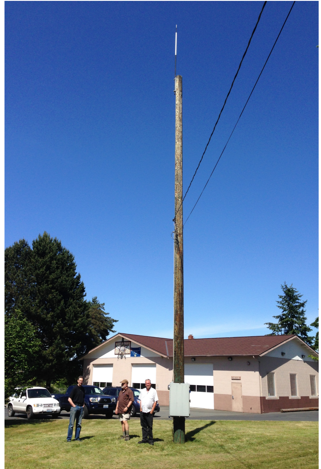
On Vashon, one of three AM transmitters is on a PSE utility pole and is powered from Fire Station.
