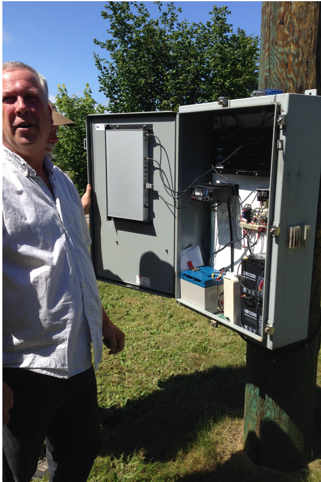
On Vashon, case contains AM transmitter gear of the type that would be desirable at Station 22 on Bainbridge.
